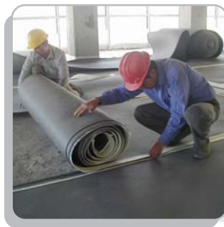
Installation of Acousti-Kal
