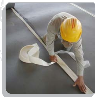
Sheet overlap blocks transmission of sound
